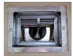
CAR damper installation with exhaust grille removed Echo Apartments (Phipps Houses)
