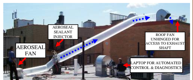
AEROSEAL System at MLK Apartments (Dunn Development)
