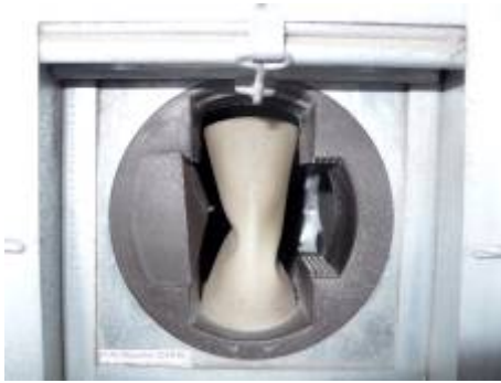
Figure 2. Constant Air Regulator (CAR-I)
