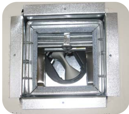
1212 MLK Apartments also incorporates Aldes Constant Air Regulator (CAR) dampers at each bathroom exhaust point. In order to regulate air flow, CAR dampers incorporate a silicone bulb that expands when the pressure drop across the damper exceeds 50 Pa.
